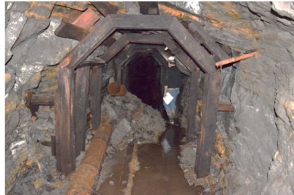
Senior Canyon Tunnel Prior to Rehabilitation
