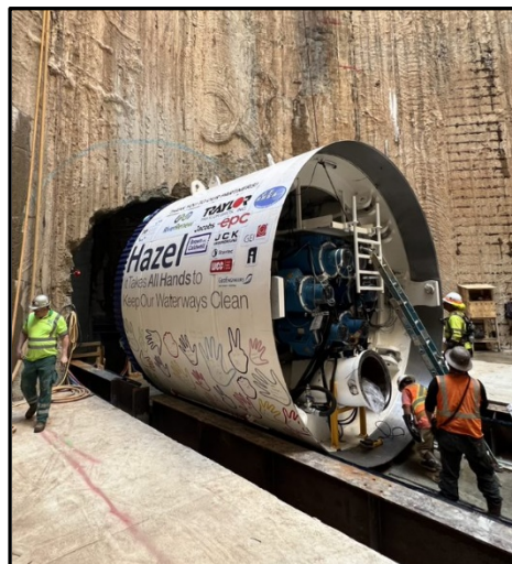
Assembling TBM at the bottom of Screening Shaft
