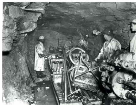
Blasting Operations for the Existing 1950's Tunnel System
