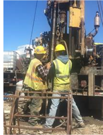
Phase I Drilling at ALCOSAN's Treatment Plant
