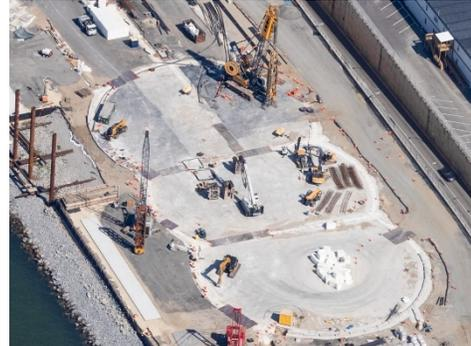
**Aerial photograph showing diaphragm wall construction on the man-made south island.**
