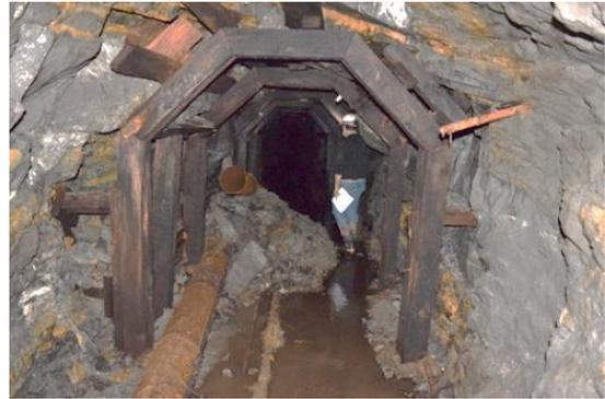
1929, the tunnel was drilled and blasted 1,555-feet into the sedimentary layers of the bedrock that form the mountains. Sometime after 1929, the tunnel was further advanced to a total length of 3,000- to 3,500-feet.
