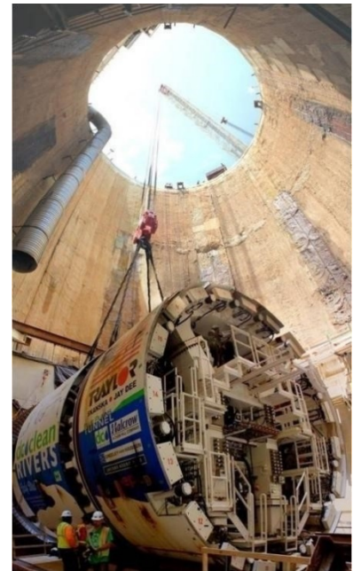
Assembly of the Blue Plains Tunnel TBM
