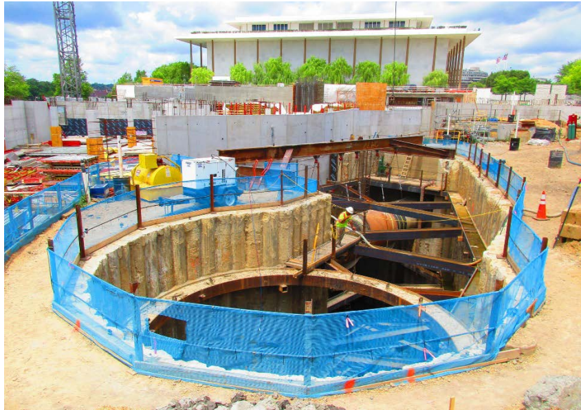
CSO-021 Project (foreground) and concurrent Kennedy Center and Expansion Project (background)
